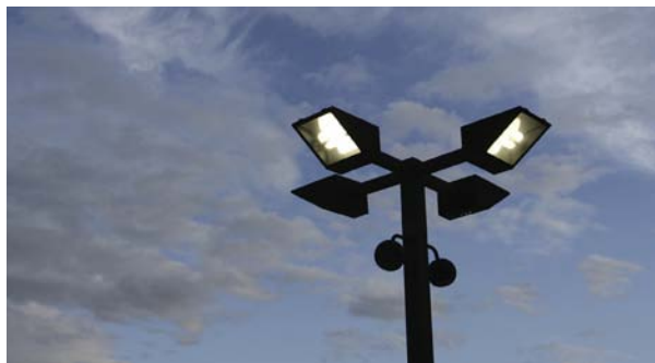
Figure 12: Exterior pole mounted lighting
