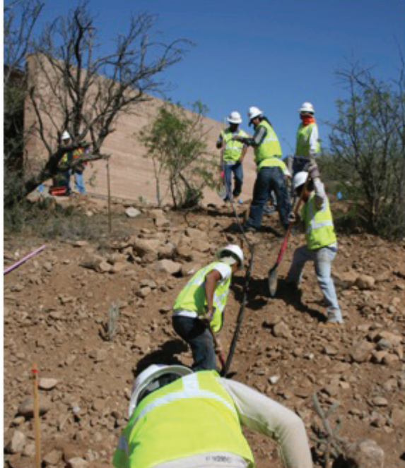
Figure 2: Crew installing drip irrigation tubing in Tucson, Arizona
