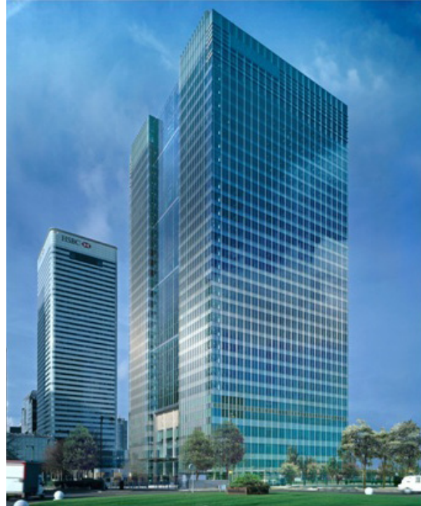
Figure 14: Exterior of Barclays global headquarters
