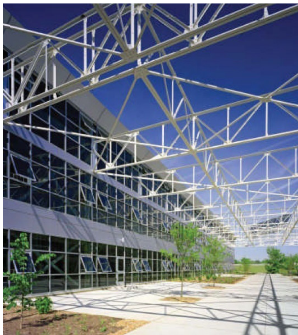
Figure 22: Exterior of Bristol-Myers Squibb research and development facility
