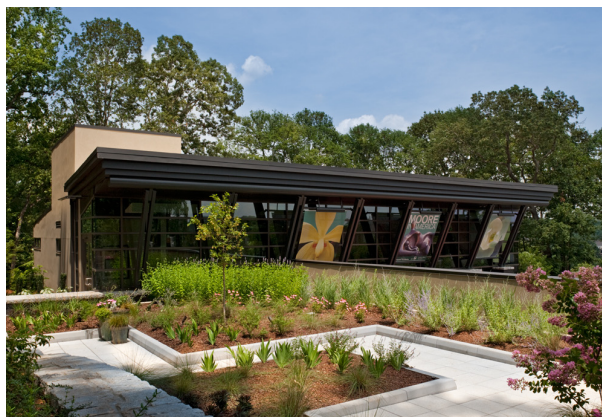
Figure 6: Green roof covering a part of the Hardin Visitor Center
