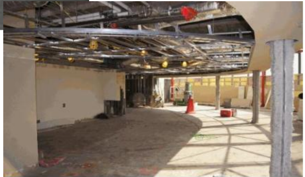
Terminal E Satellite - Lower Level Club Framing & Utilities
